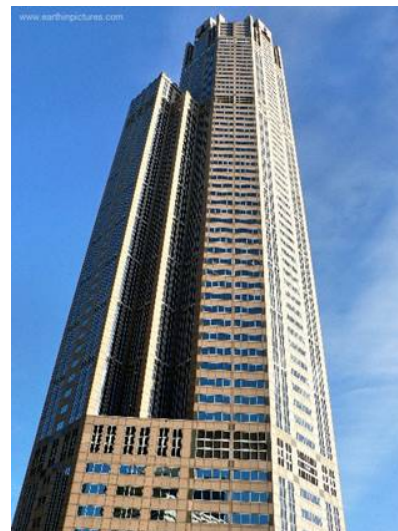
Figura 3. South Wacker Drive
